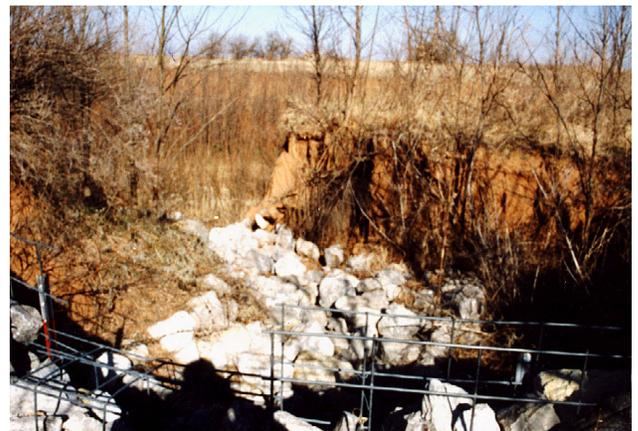
Figure 11c. Tree growth below upper gabion, in the first winter following treatment. The larger trees are 5 years old.
