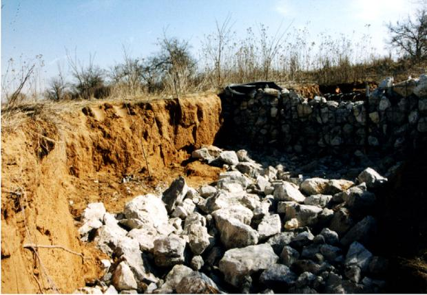
Figure 10b. Completed upper gabion and upper part of chute
