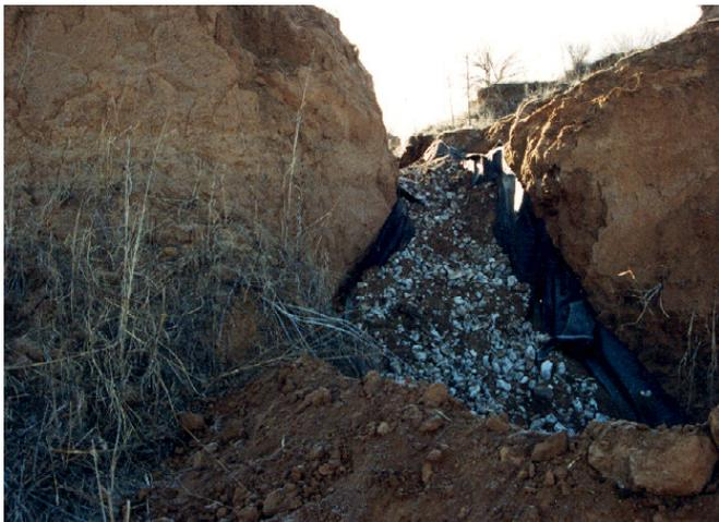
Figure 9a. Chute with geotextile fabric and small rock placed
