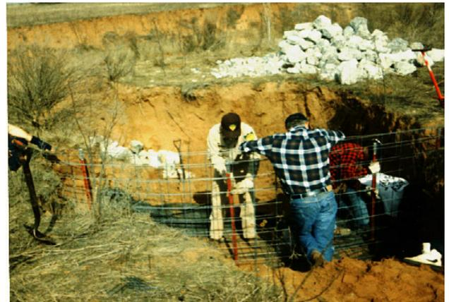
Figure 10a. Constructing the upper gabion
