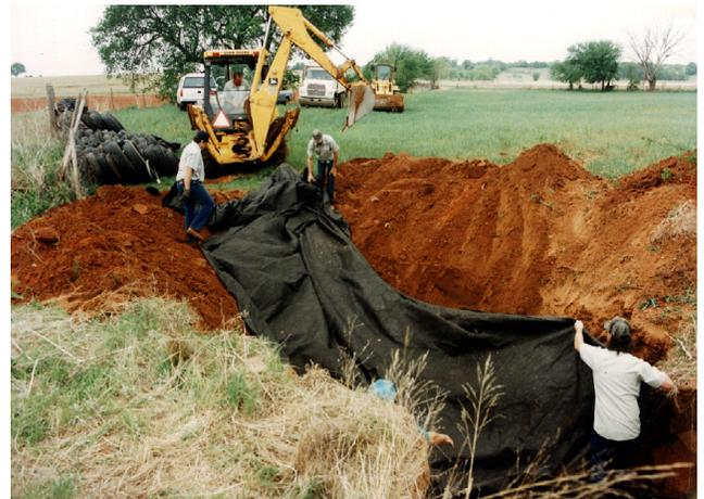
Figure 15c. Applying the geotextile fabric
