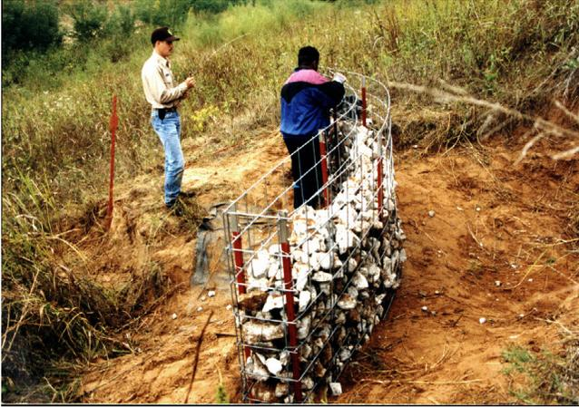
(Above) Lower gabion on Tillman County gully during construction in 1999
