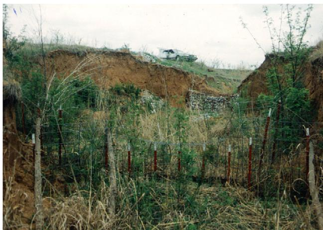
Figure 13c. Gully bottom control below the Example 2 drop-structure, constructed by placing cattle panels next to the gully sides and across the bottom. Photo was taken in the first growing season.
