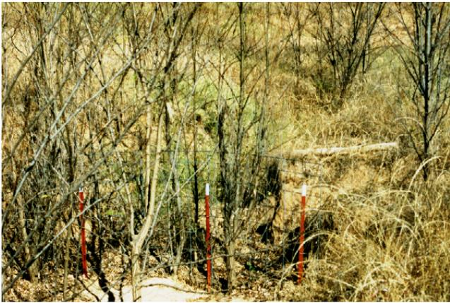
Figure 5. Lower part of a small gully on the Tillman County system, controlled by installing a curved cattle panel with T-posts and planting black locust trees
