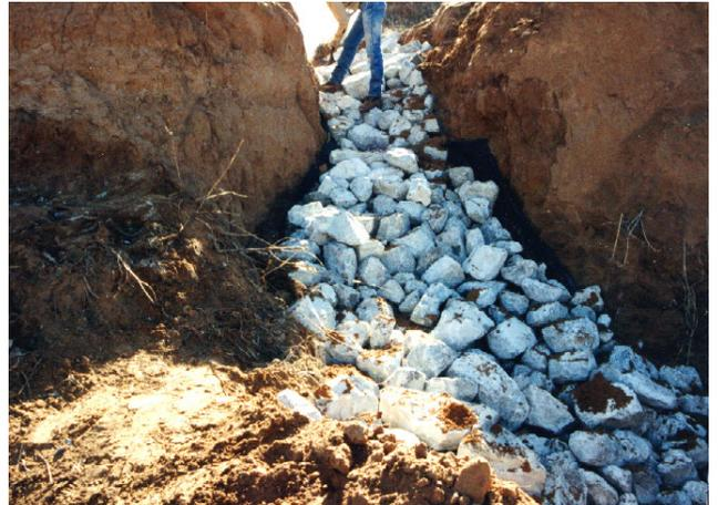
Figure 9b. Completed chute with large rock placed
