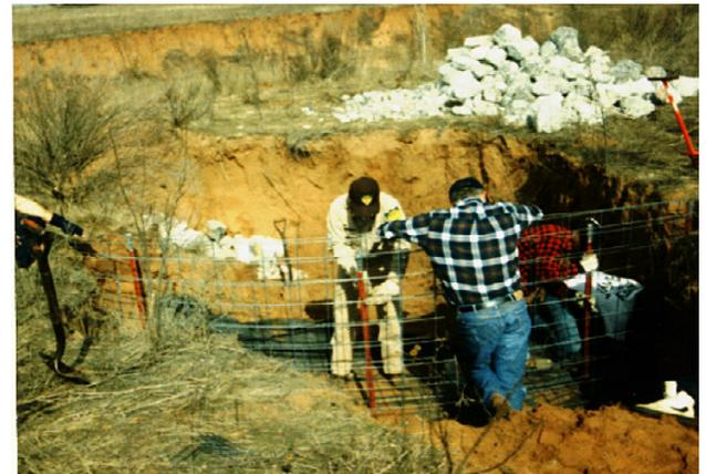
Figure 10a. Constructing the upper gabion
