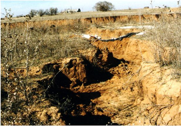
Figure 10c. Upper gully area and completed upper gabion. Note geotextile fabric and soil cover on the upper side of the gabion.
