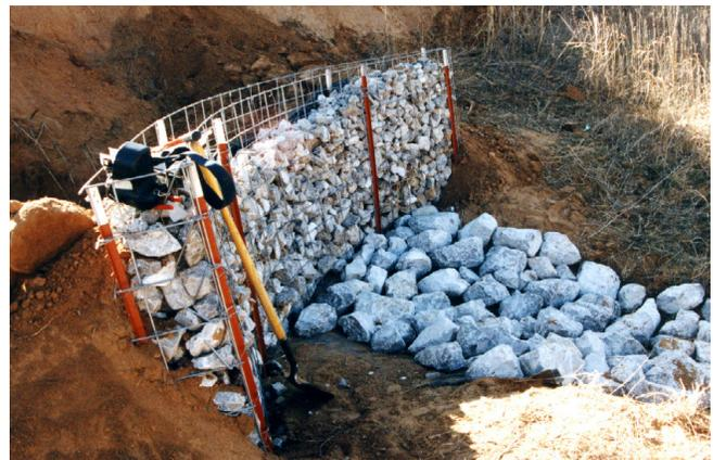
Figure 8b. Completed lower gabion with apron
