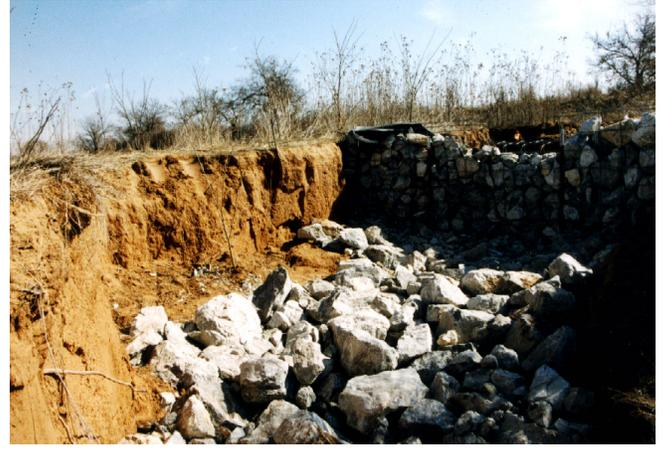
(Above) Upper gabion on Tillman County gully during construction in 1999
