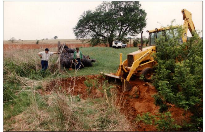
Figure 15a. First steps in construction on Example 3 were to shape and slope the upper gully area (note black locust saplings)
