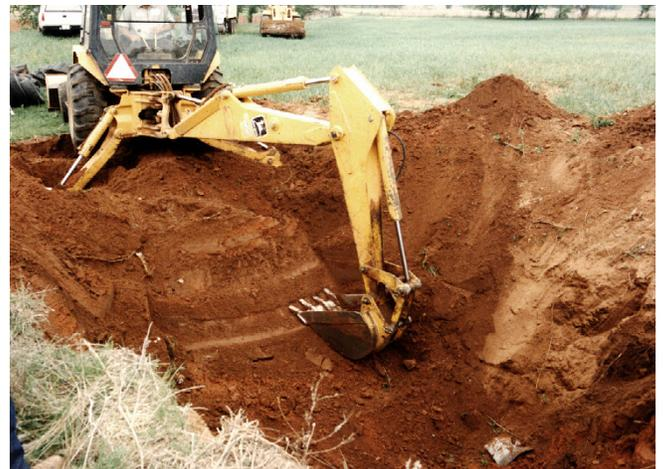
Figure 15b. The backhoe was used for final shaping
