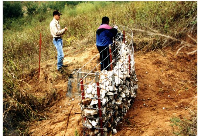
Figure 8a. Constructing the lower gabion drop structure
