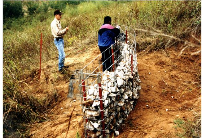
Figure 8a. Constructing the lower gabion drop structure
