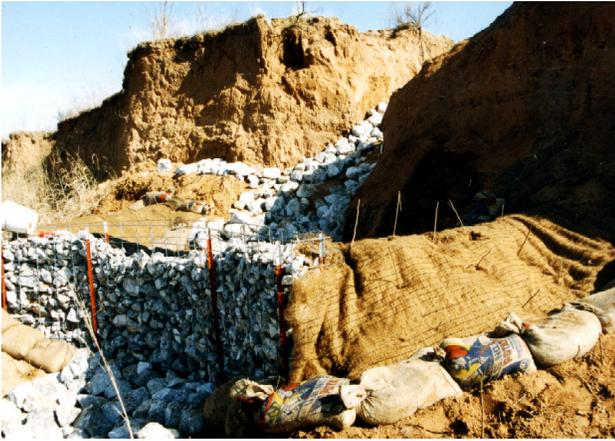
Figure 8c. Lower gabion with wing walls completed and black locust seedlings planted
