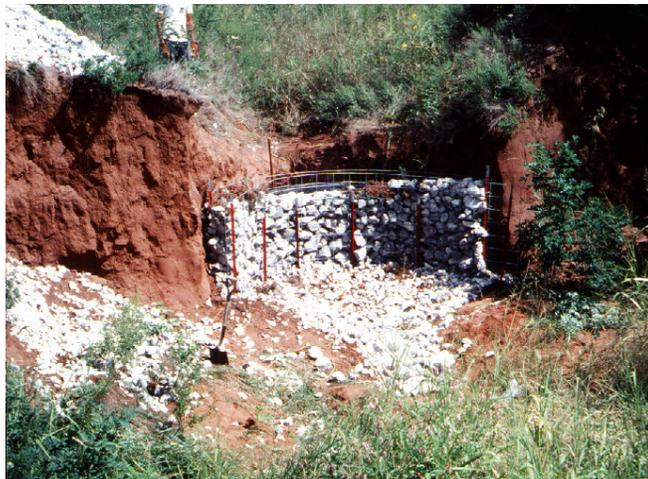
Figure 13b. Completed gabion drop-structure and apron
