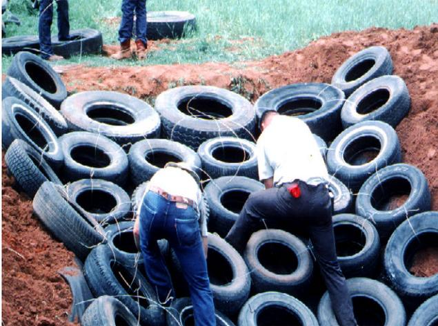
Figure 15d. Placing and wiring the tires
