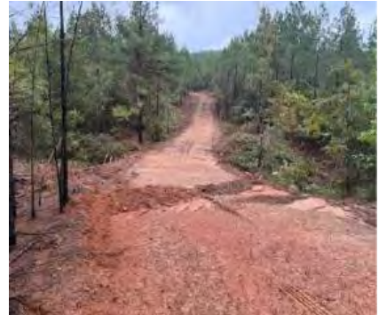
Example of road construction with water diversion practices in Latimer County
